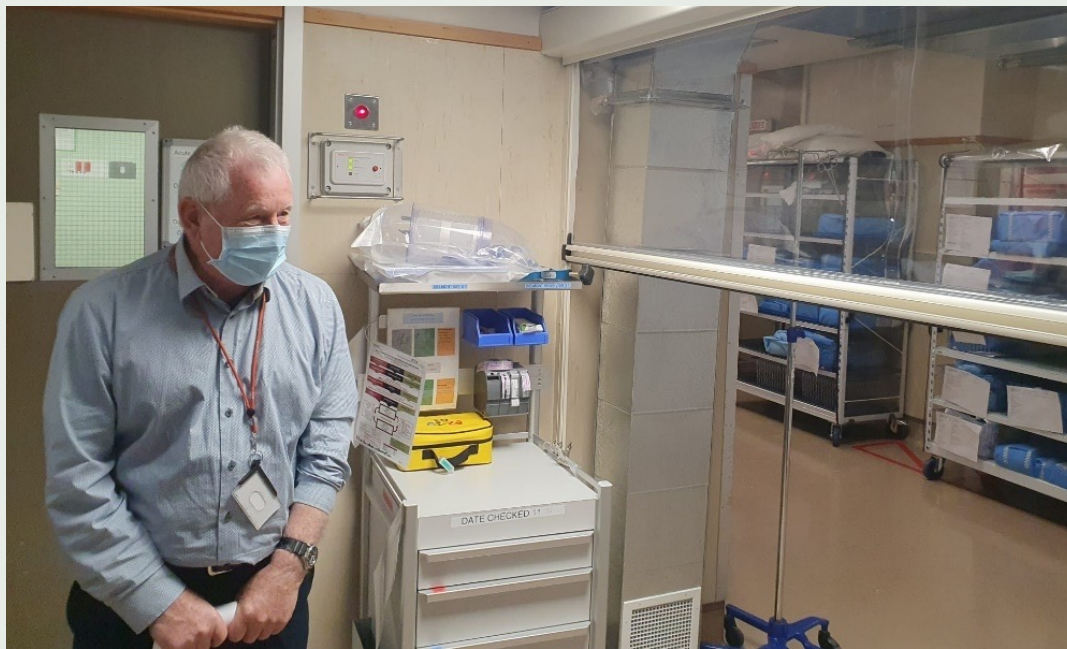
Palmerston North Hospital engineer with the pull-down screen used to create a separate 'red' zone in the operating theatre.
